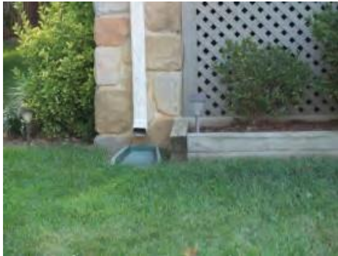
Figure 0.33 Simple Rooftop Disconnection Photo: Center for Watershed Protection
