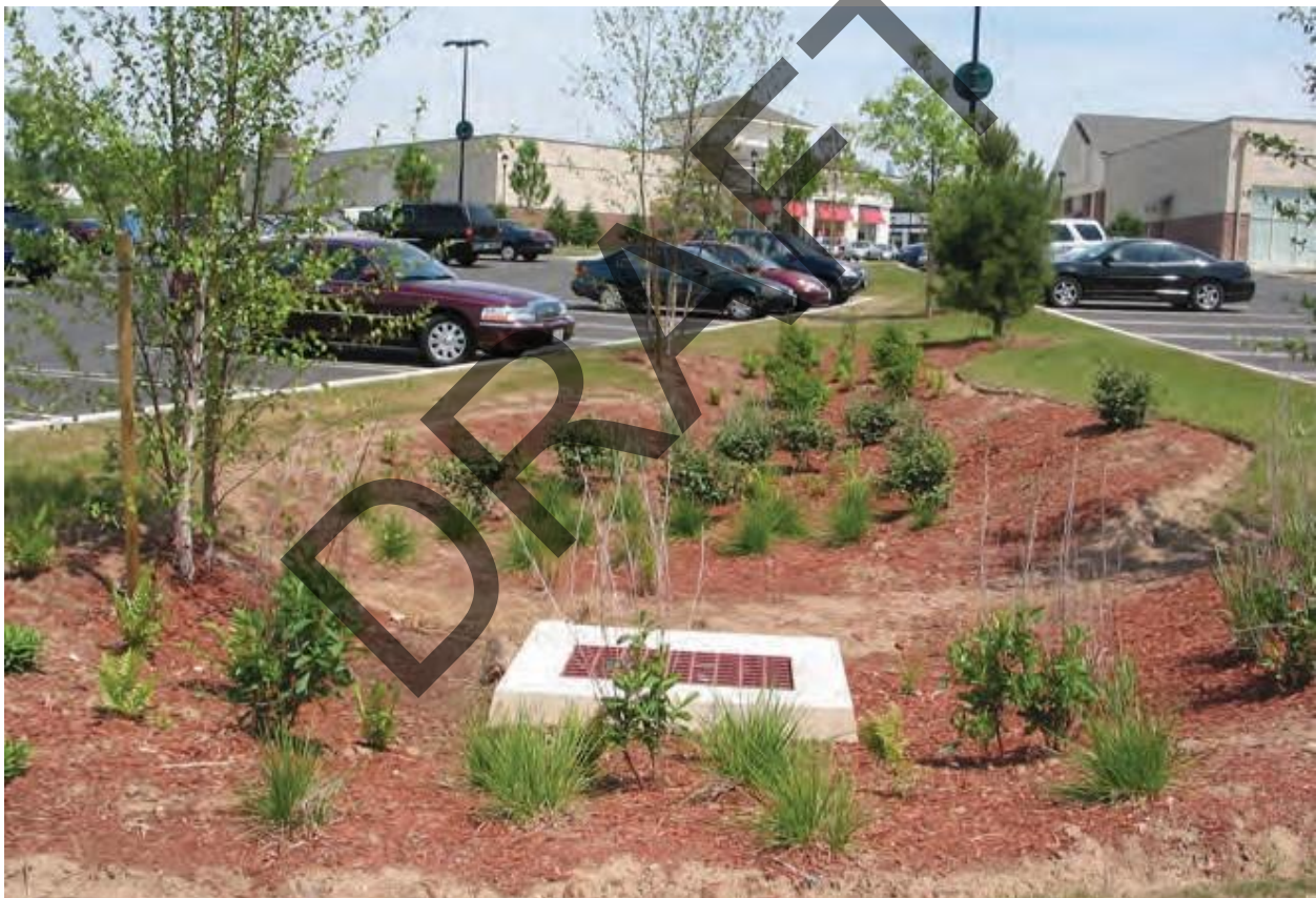
Figure 0.1 Bioretention in Parking Lot Photo: Center for Watershed Protection
