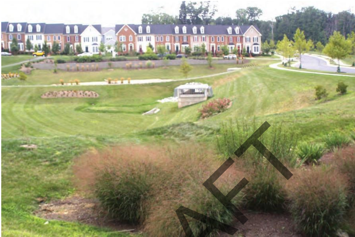
Figure 0.46 Dry Extended Detention Pond (Photo: Center for Watershed Protection)
