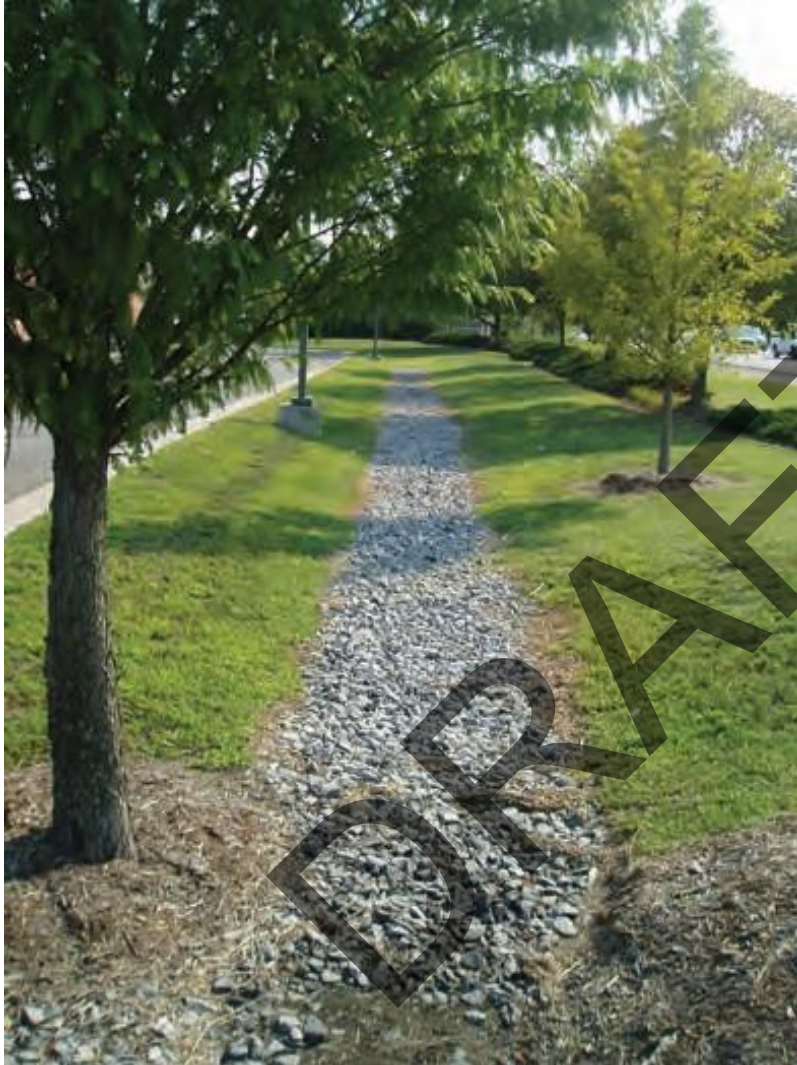
Figure 0.17 Infiltration in Median Strip
